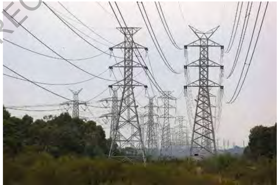
Transmission lines and towers near Melbourne
